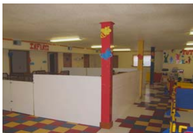
Figure 12: Load bearing columns required to create a classroom-sized space in a structure built for another purpose. (Photo Source: Carl Sussman)
